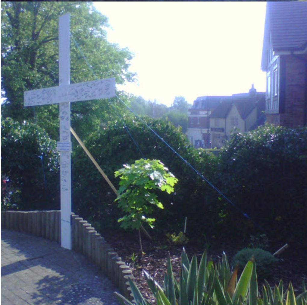
Trinity Church Knebworth used guy ropes at the back pulling against a wooden strut, as suggested in the leaflet. Names were added after the cross was put up.
