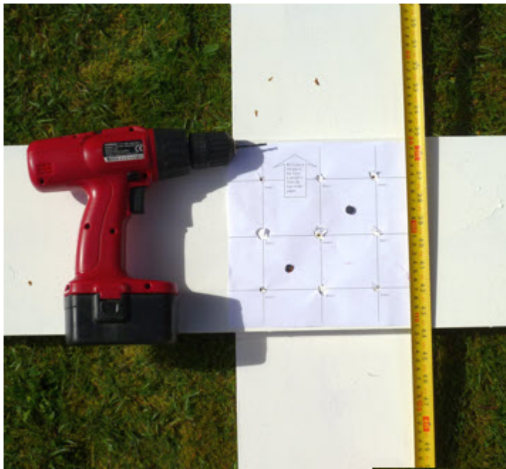
The template in place, held by drawing pins, before the drilling of the holes and screws were put in at front of the cross ( Left )
